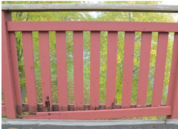
Figure 5.38. Bad detail, railing panel of spruce, one layer of primer with fungicide, two layers of paint, severe decay in the lower part due to water trap between pickets and lower panel rail.
