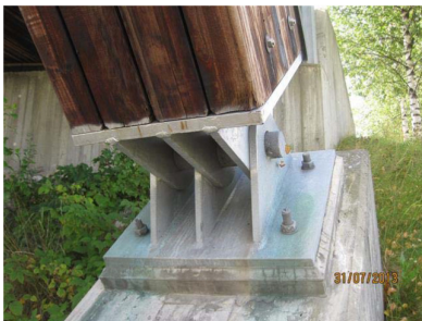
Figure 5.30. Bad detail, copper ions from copper fitting runs down to the underlying joint and corrodes the zinc coating.
