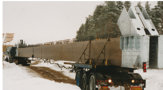
Figure 3.15 Transporting a timber beam member for composite deck
