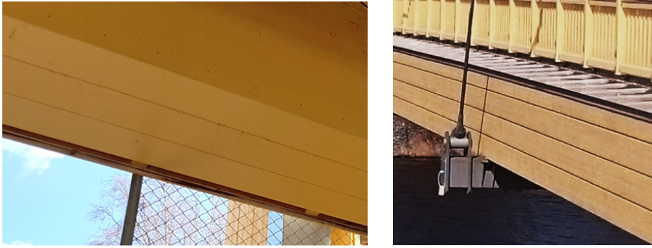
Figure 5.21. Good design. Left: Painted glulam beam with painted cladding of ventilated horizontal wood panel on vertical battens on the outside. Right: The outside of the cladding and on top of the beam is a ventilated steel plate.
