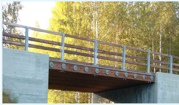
Figure 3.8 Pre-stressed slab bridge
