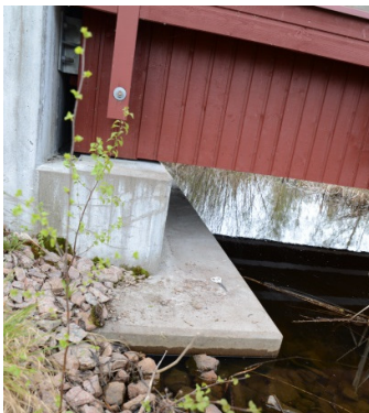
Figure 5.5. Bad detail, new bridge with risk of gravel and dirt to be collected on the abutment.
