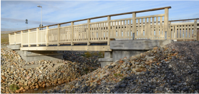
Figure 4.27. Pedestrian bridge with SLT deck, Umeå, Pousette and Fjellström (2016).
