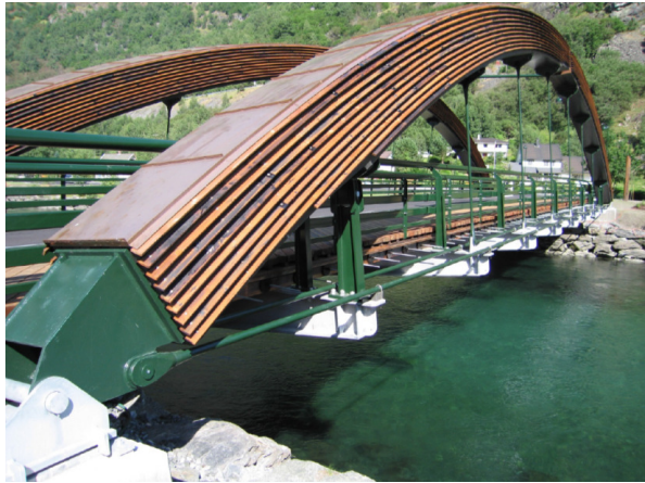
Figure 3.5 Fretheim bridge, span 38 m, with three-hinged glulam arches, stress-laminated timber deck, steel hangers, steel cross-beams and no horizontal wind truss between arches. Photo: Sweco Norway AS
