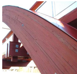
Figure 5.27 Arch bridges. In A the arch was unprotected but painted and had several cracks. In B the top of the arch was protected with a steel cover, but the sides were still unprotected. In C the sides were covered with a ventilated cladding of painted plywood sheets. The growth of cracks should then be significantly reduced and water cannot penetrate into the cracks.
