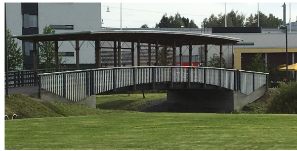
Figure 3.11 Timber bridge equipped with canopy
