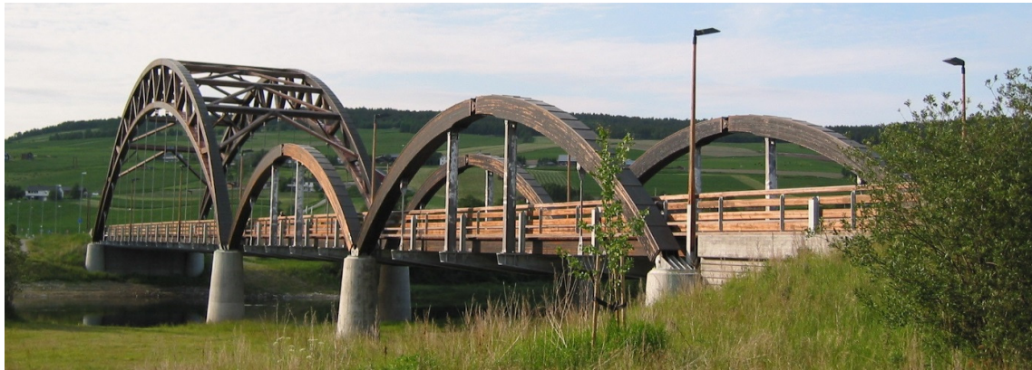
Figure 3.21 Tynset bridge, Norway (photo: K. Bell)
