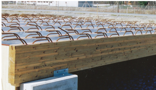
Figure 3.14 Timber beams installed before casting of the concrete slab
