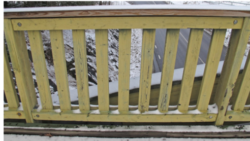
Figure 5.39. Good design, railing panel of treated pine, NTR class A, two layers of primer with fungicide, two layers of paint, paint erosion on all parts but no visible signs of decay.
