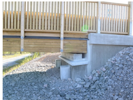
Figure 5.6. Good design, new bridge with good ventilation at abutment.
