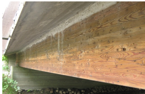
Figure 3.13 Timber beam and concrete slab
