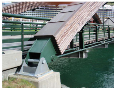
Figure 5.31. Good design, water from copper fitting is taken out to the side before it reaches the bottom section.
