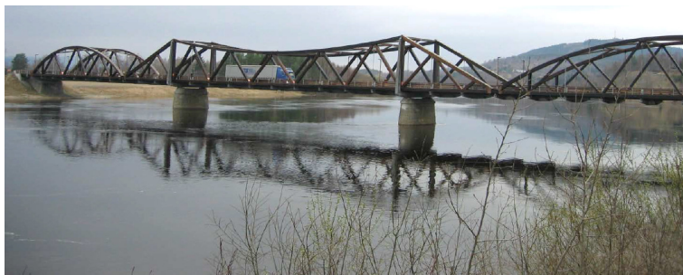
Figure 3.3 Flisa bridge, Norway, truss with longest span of 70 m. Photo: K. A. Malo
