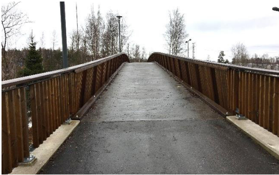
Figure 4.1 Asphalt cover on the timber deck
