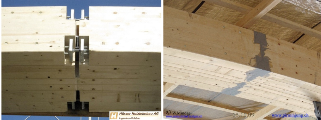
Figure 3.57 Example of application of glued-in rods in the apex of an arch bridge, Kirchenbrücke, 2009, Switzerland, source: www.swiss-timber-bridges.ch
