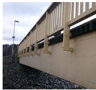
Figure 6.3. Painted beam bridge (Vaxholm, Sweden)
