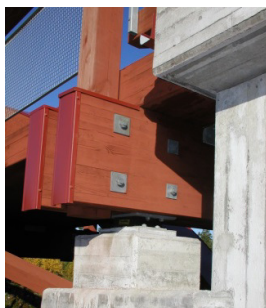
Figure 6.2. Cross beam painted red (Falun, Sweden)
