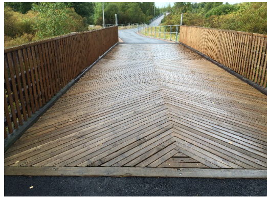
Figure 4.3 Diagonally nailed plank deck
