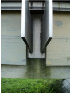
Figure 5.34. Bad detail, railing post is designed so that water is directed towards the deck edge.
