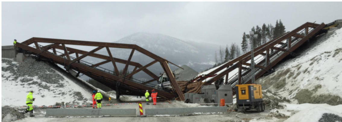
Figure 3.50 Perkolo bridge hours after the collapse (Photo: R. Abrahamsen)
