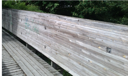
Figure 5.18. Bad design, large salt-impregnated glulam beams of pedestrian bridge without cladding, with typical cracks and delamination.
