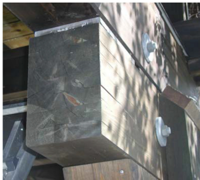
Figure 5.19. Bad detail, no cover of end grain and typical cracks and delamination.
