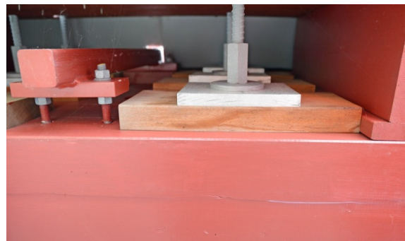
Figure 5.10. Good design, only small amounts of water follows the railing posts but it does not affect the moisture content in the deck.
