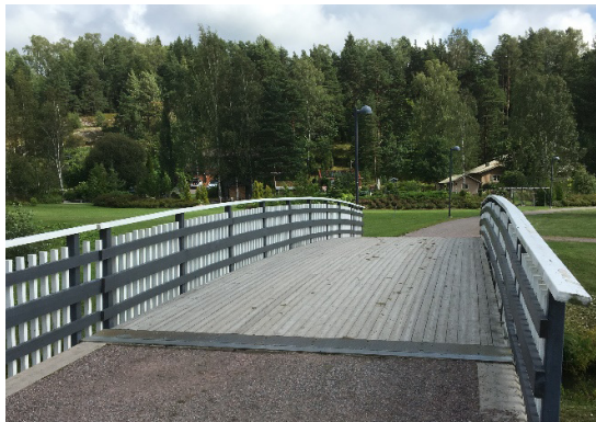
Figure 4.2 Longitudinal nailed plank deck
