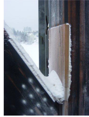
Figure 5.26. Good design, metal fitting protects the slot.
