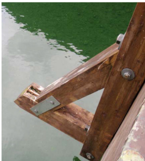
Figure 5.32. Bad detail, railing with no constructive protection, and water flows along diagonal and decay has occurred in lower part.
