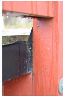
Figure 5.37. Good design, sheet metal between bridge deck and railing post protecting from water and no decay in wooden distance or in railing post.
