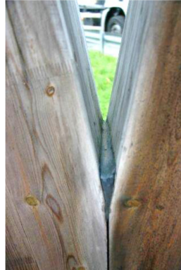
Figure 5.25. Bad detail, sealant creates moisture pocket after some years.
