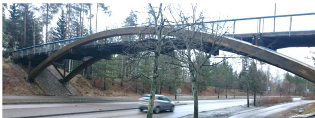
Figure 1.3 Timber arch bridge, Finland
