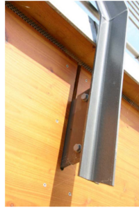
Figure 5.35. Good design, railing post is extended so that the lower part serves as a dripping nose.
