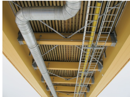
Figure 5.23. Good design, tube and cables are installed under the deck, protected from moisture and will not moisten the beams.
