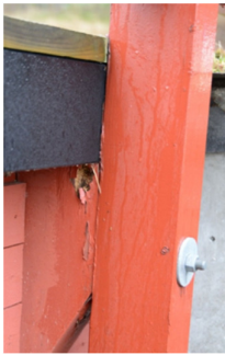
Figure 5.36. Bad detail, railing post attachment, sheet metal cladding is missing and wooden distance have severe decay damage.
