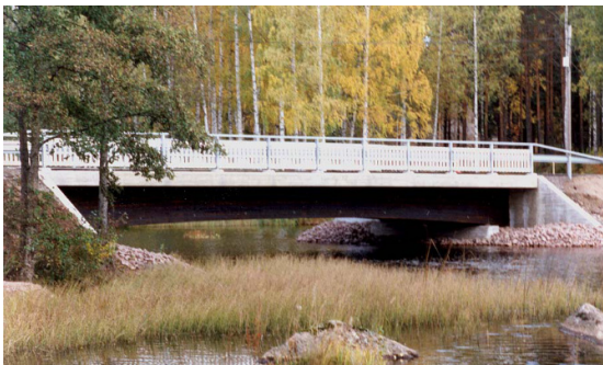
Figure 3.12 Timber-concrete bridge
