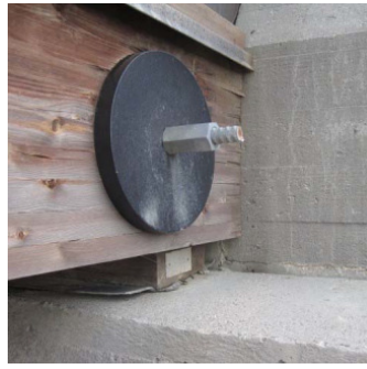
Figure 5.8. Good design, sill beam is drawn in under the deck, but still foundation ledge protrudes.
