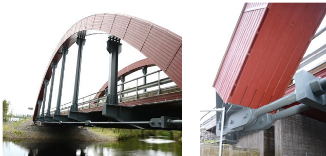
Figure 6.1. Arch protected with ventilated cladding of boards on the sides and steel hood on top, arch and cladding painted red (Gislaved, Sweden). Right: Underside of arch at support.
