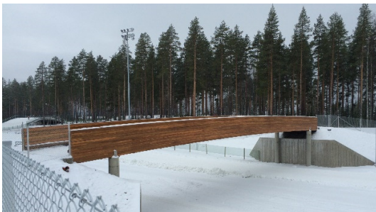
Figure 3.10 Cantilever beam bridge
