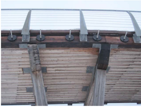
Figure 5.11. Bad detail, running water under the deck because edge detail does not work, possibly due to a joint.
