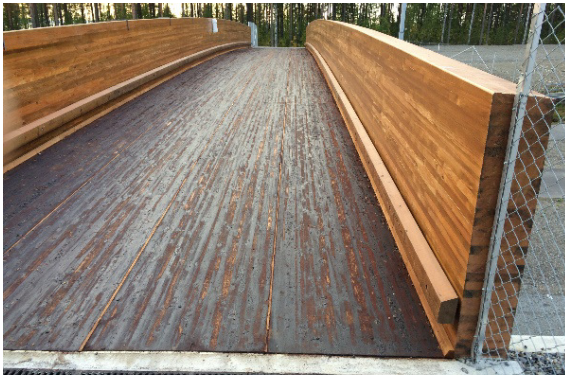
Figure 4.32 Longitudinal glulam deck.
