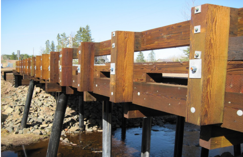
Figure 4.30. Example of a Spike-laminated deck bridge in Minnesota (USA).
