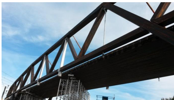
Figure 1.2 Construction of timber truss bridge, Norway
