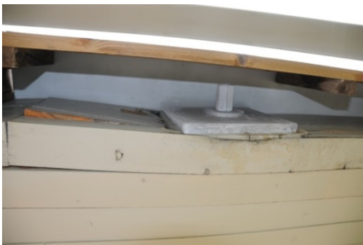
Figure 5.9. Bad detail, high moisture contents, the leakage came from inadequate execution at the edge and the rail posts.
