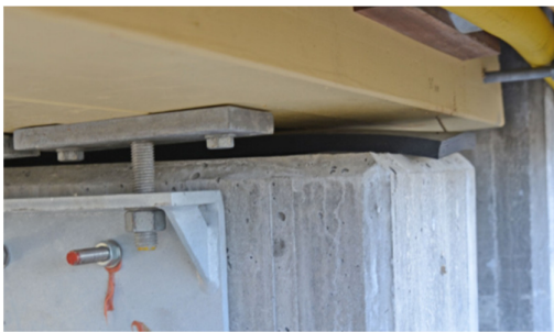
Figure 4.28. Cupping in every corner of the deck, Pousette and Fjellström (2016).
