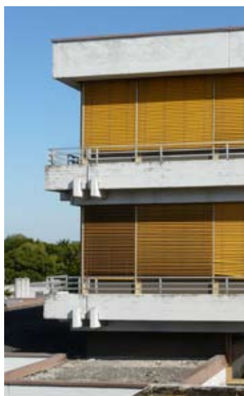
189. Before modernisation - concrete balconies
