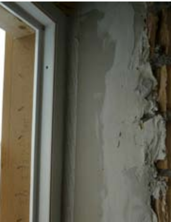
123. Airtight joint at window reveal with a double layer gypsum fibre board
