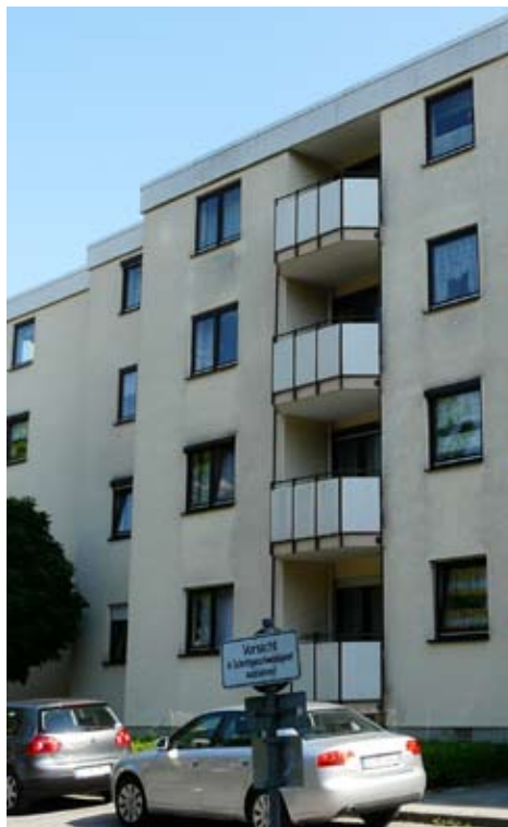
55. Partly cantilevered slab
