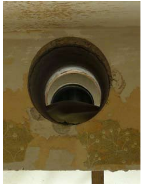
179. Pipe lead through above a window
