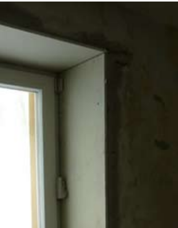
123. Airtight joint at window reveal with a double layer gypsum fibre board
