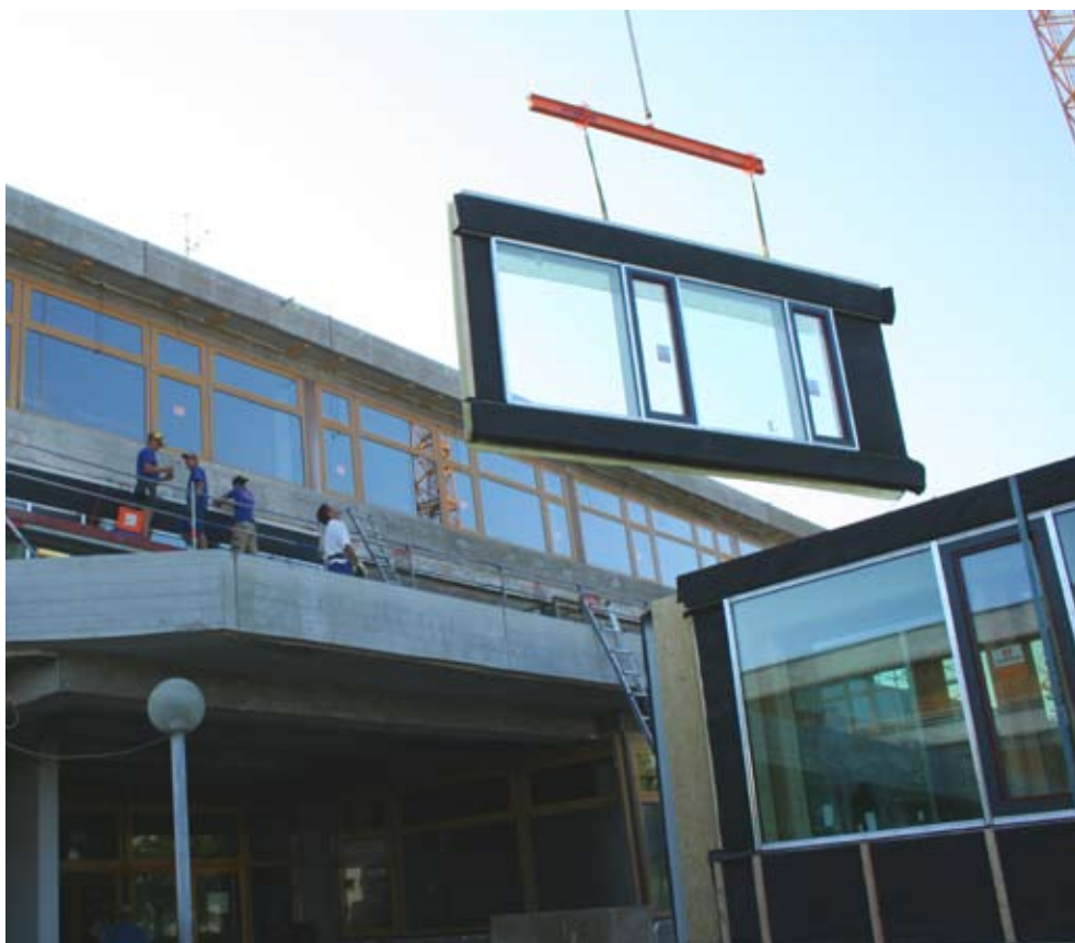
193. Mounting of TES elements
