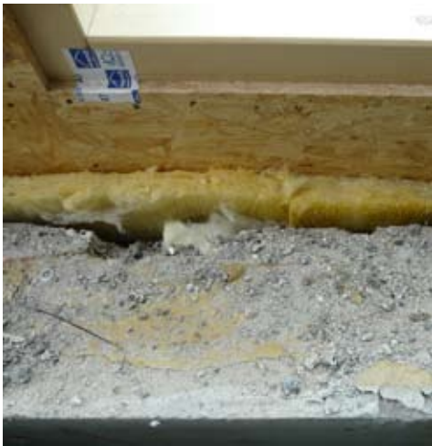
102. Element joint at sill
