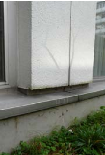
34. Joint in concrete skeleton structure
