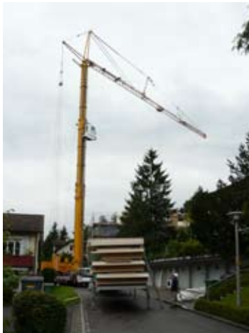
167. Transport of lying elements on bridge plate.
