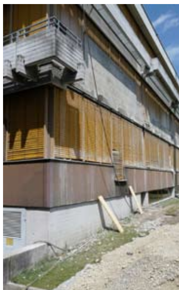
190. Demolition of balconies and old façade
