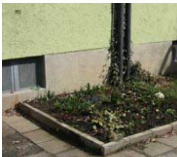
20. Base with cellar window
