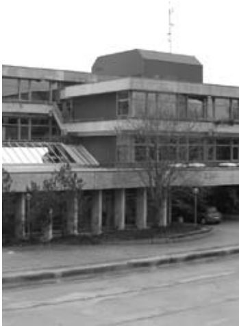
187. Existing building entrance
