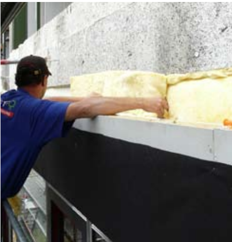
101. Fixation of adaption layer on the existing wall. Depicted here is a Heraklith surface, Real-schule Buchloe
