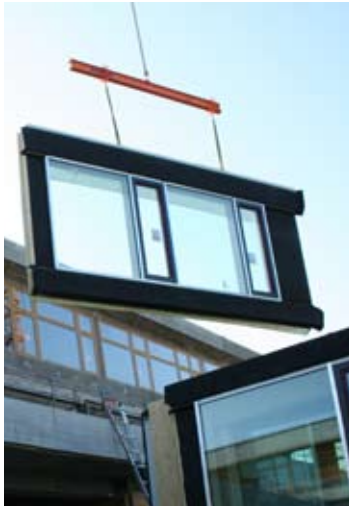
8. Prefabricated façade element assembly at Realschule Buchloe.
