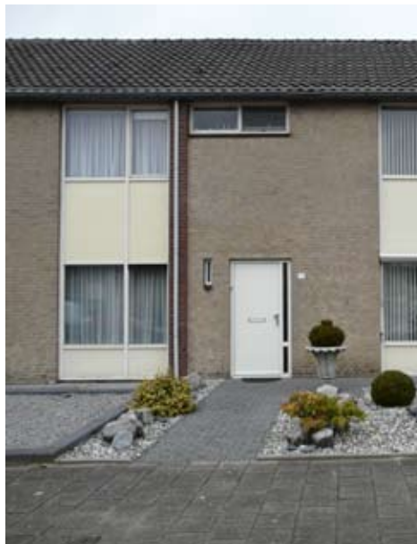
44. Double layered brick masonry with timber framed window element, 10 cm, poor insulation standard, NL-Roosendaal
