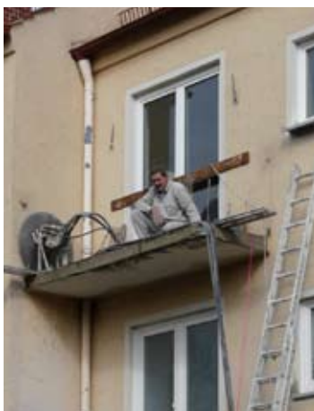
57. Cutting off balcony slab
