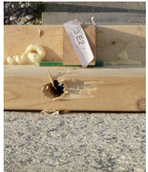
113. Drilled hole for filling hose.
