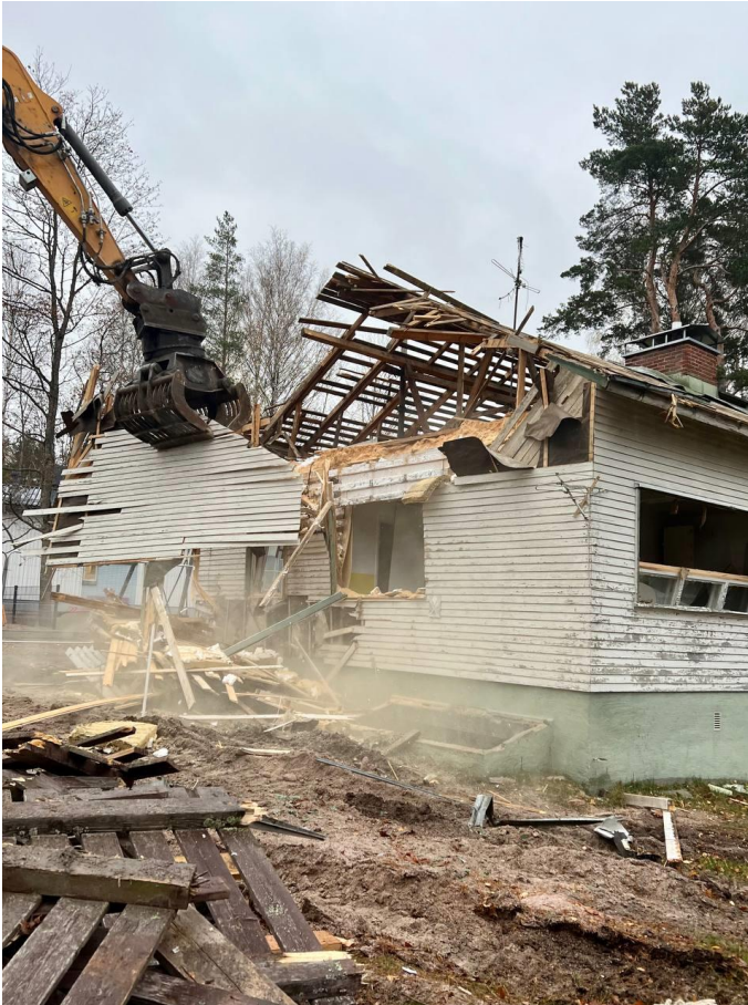
Figure 4.3 Heavy demolition phase of a wooden building located in Espoo, Finland.
