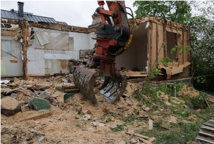
Figure 4.4 Heavy demolition phase of a residential house located in Jyväskylä, Finland.
